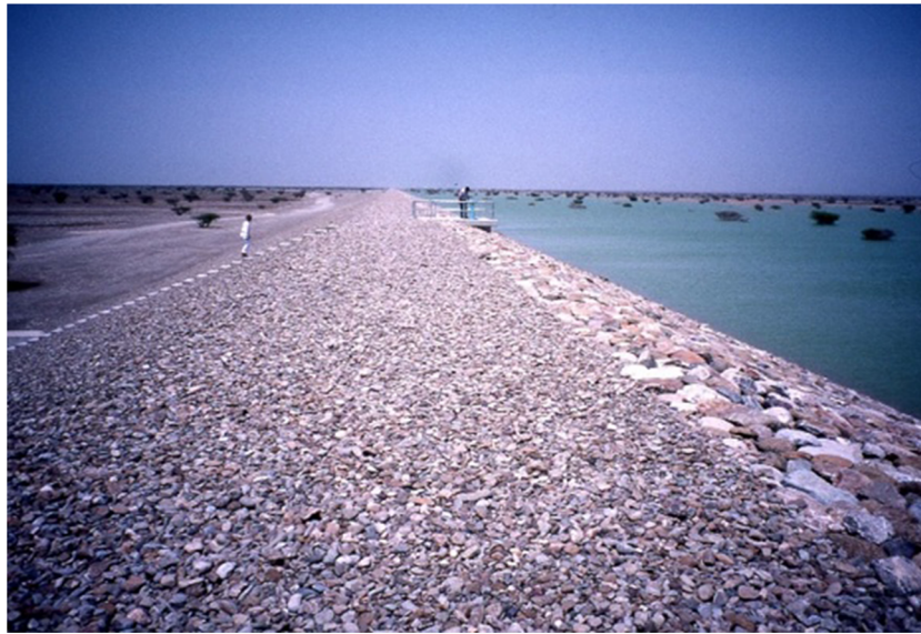
Fig. 6 Ahin recharge dam on the Batinah Plain, Oman, constructed in 1994, is a large dam (crest length 5,640 m, crest height 8 m) with a detention capacity of 6.8 Mm 3 . This is one of the 43 recharge dams, with an aggregated capacity of 95 Mm 3 constructed in Oman during the period 1985–2011 (Oman MRMWR 2012). Their purpose is to enhance aquifer recharge primarily to support irrigation; and also to protect the
