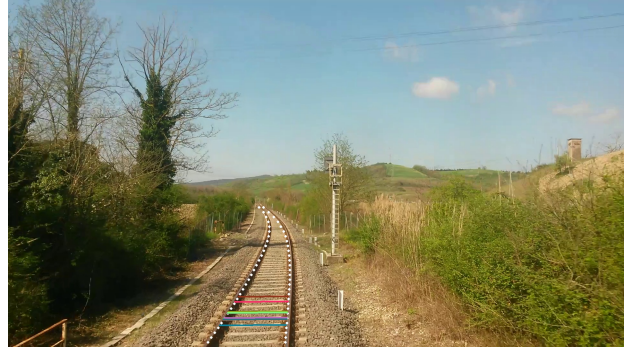
Fig. 3. Tracking of the rails and railroad ties in order to achieve their line fitting. Small rail elements within a frame have been subsequently detected using a template matching algorithm to obtain the whole rail profile. For each template the blue markers indicate the position of lower left corner. The lines approximating the rails are gathered by a polynomial fitting of the lowest 15 templates.
